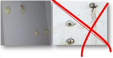
Bolts on the doors may damage the surface of K-Flex. Cover the sharp edges of the bolts with silicon and cover the doors with thick carton boards.
